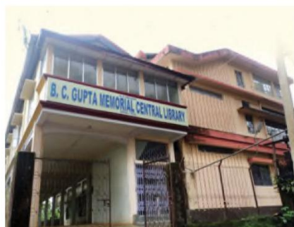
Central Library Building
